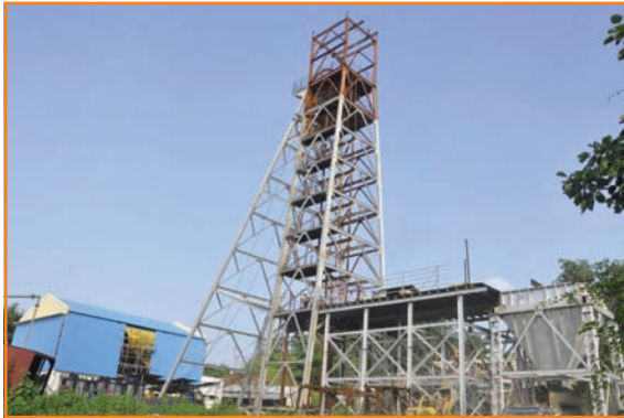
2 nd Vertical Shaft at Chikla mine
