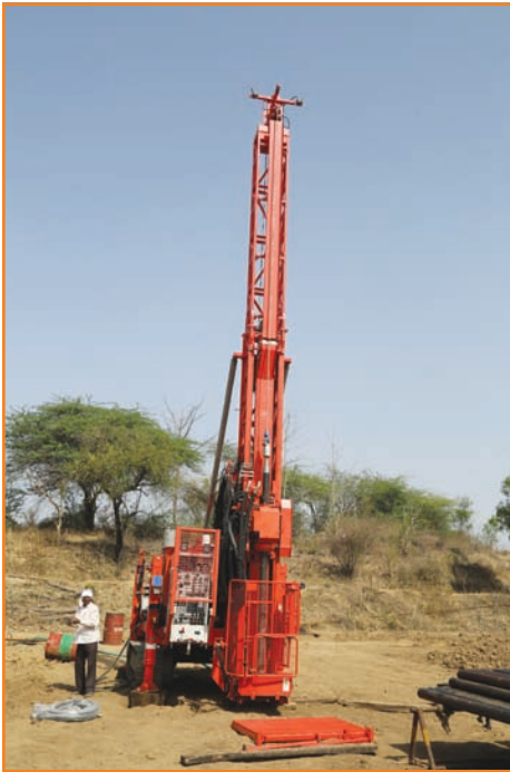
Exploration Drilling Machine Installed at MOIL'S Mine
