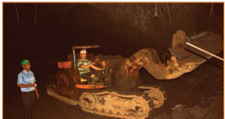
Underground Single Boomer Crawler
